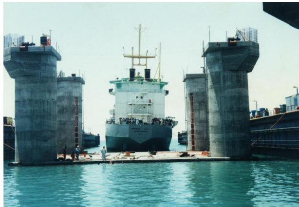
Fig.9: The caisson is brought out of the basin by a tugboat
