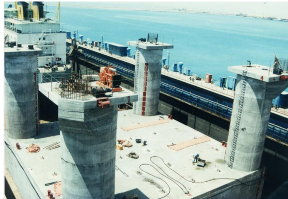
Fig.8: the caisson floating in a basin in “Persian Gulf Shipbuilding Co”
