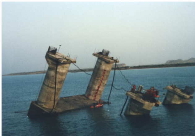
Fig.11: the drowning caisson
