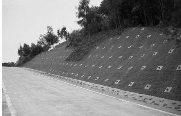
Fig 2: Example of wall by nailing
