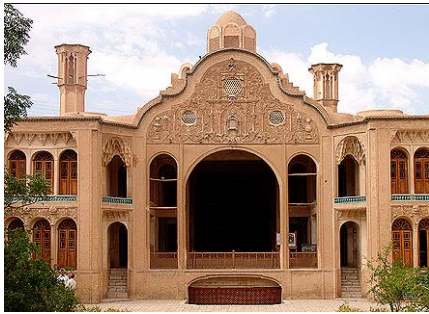
Fig 1: Summer house of Borojerdiha house in Kashan
