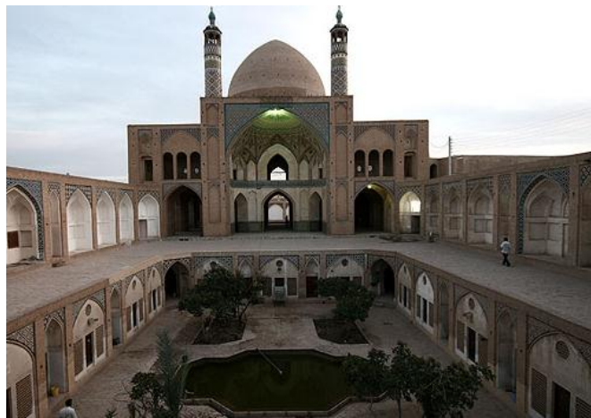
Fig 1: Garden cavity Aga Bozoeg mosque and school in Kashan
